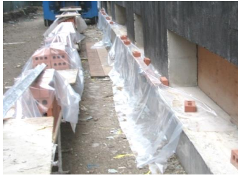
Figure 6. Photo of end of day protection
