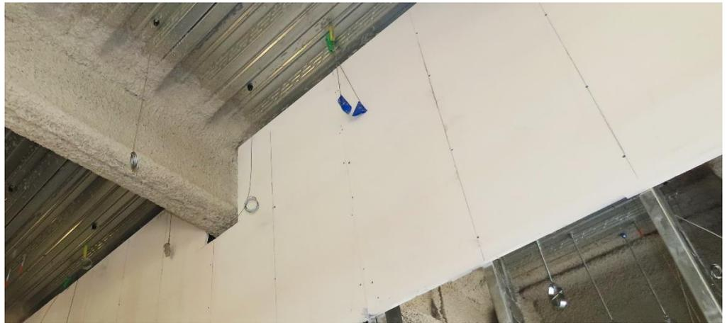
***This clarification to the Limiting Height Tables will likely reduce the allowable heights and potentially increase our stud gauge, spacing, top track type, and/or width of framing to meet the allowable heights.***
